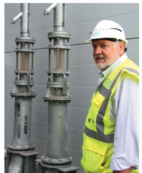
–A practical feature I like are the visual control points, like here on these pneumatic conveyors. It's a simple but great complement to computer screens, easy for anyone walking around the plant to spot a potential hitch, said Andrew Wood.
