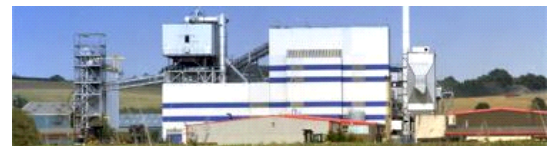
EPR - Fibrogen power plant.
